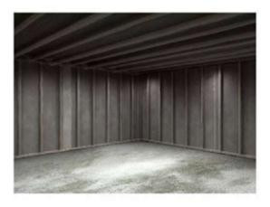
If this is a remodeling project, it is OK to wrap the existing studs in the room as shown, in a similar fashion to ceiling joists. Make sure the vapor barrier is on the warm side of the wine cellar, meaning the exterior cellar wall.
